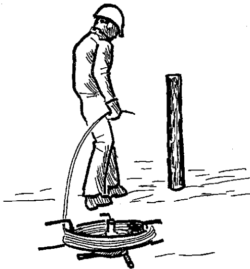
A rotating payout reel is used to string the guide wire.
